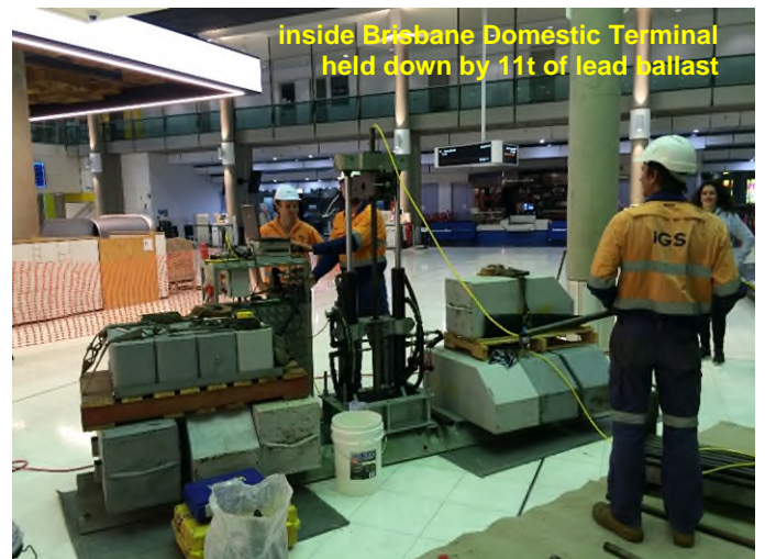
on the Brisbane Airport Link Tunnel – horizontal tests to 38m+
